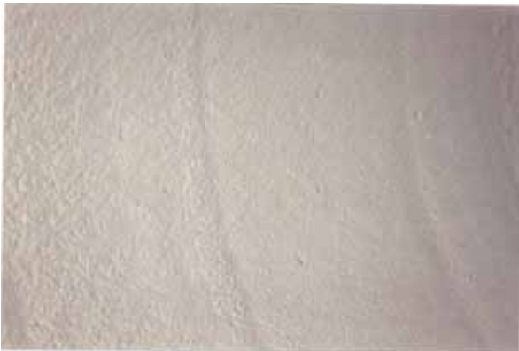
Fig. 1 Internal surface of aqueduct’s metal pipe after shotcreting with PLASTCRETE mortar
