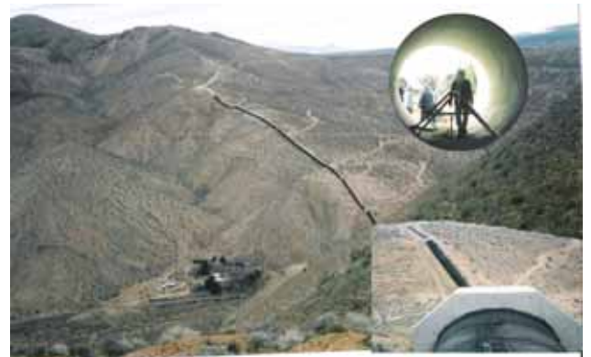
Fig 2. Metal aqueduct \approx \varnothing 3.5 m and length of 129 km (80 miles) experiences salient water hammers up to 50 bars. Shotcreting works are being continued.
