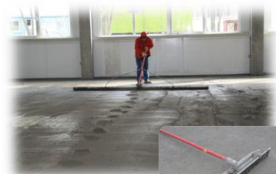
Application KF-G remedial slurry
